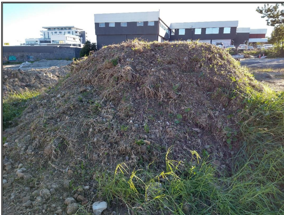
Figure 6: Stockpile of stripped surface fill comprising some brick and concrete, 9 June 2022.
