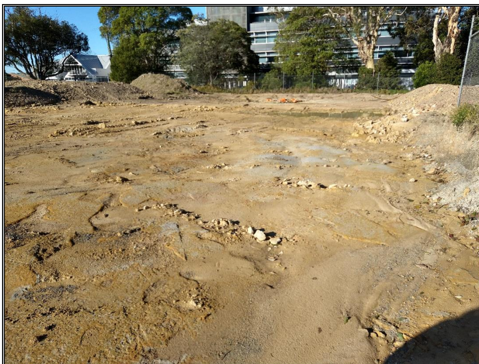
Figure 7: Exposed natural soils in south western portion and surrounding stockpiles of stripped fill materials, looking south west 9 June 2022.
