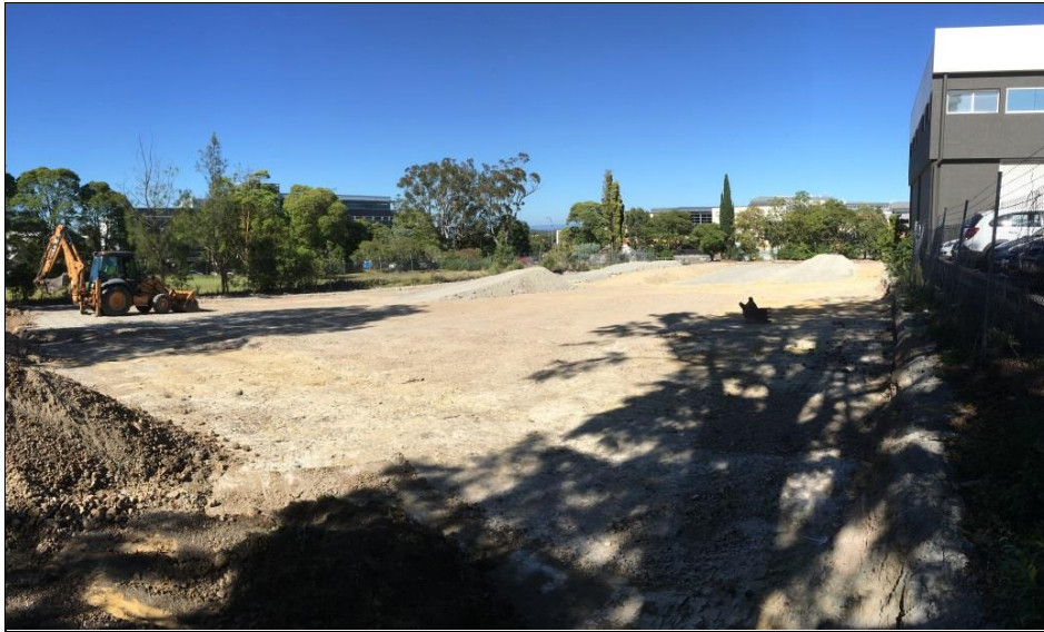
Figure 2: Majority of the remediated site, with the consolidated stockpiles of the excavated upper 'clean' fill and deeper fill within the RAC in the background, looking south west (11 December 2017).
